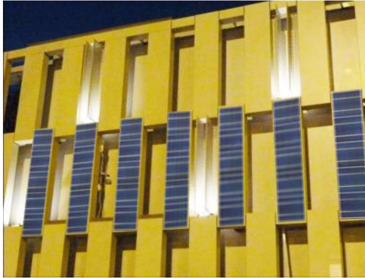
Figure 30: Proposed BIPV on South-Facing 'Veil' Façade [Photo credit: HLB Lighting, Inc., 'veil' mock-up]
